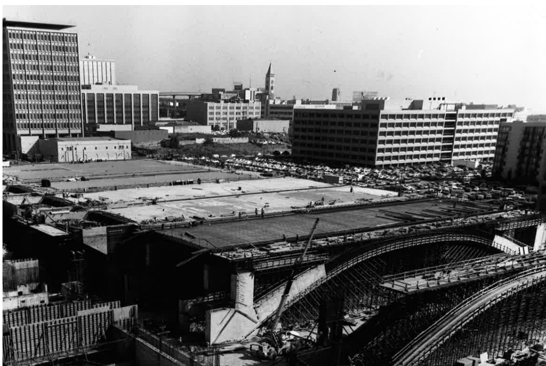
The Moscone Center under construction prior to 1981, showing the distinctive arches of its underground column-free hall.
