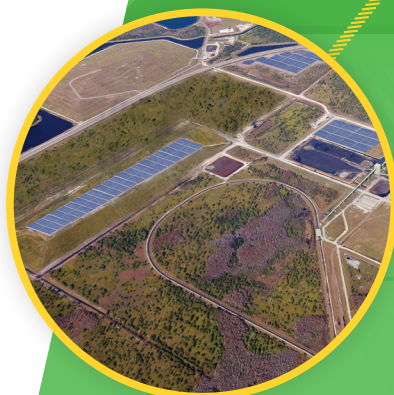
KENNETH P. KSIONEK COMMUNITY SOLAR FARM 13 MW
