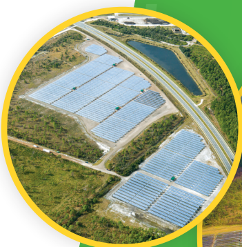
SOLAR FARM I 6 MW
