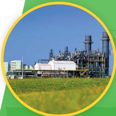
UNITS A & B NATURAL GAS 940 MW
