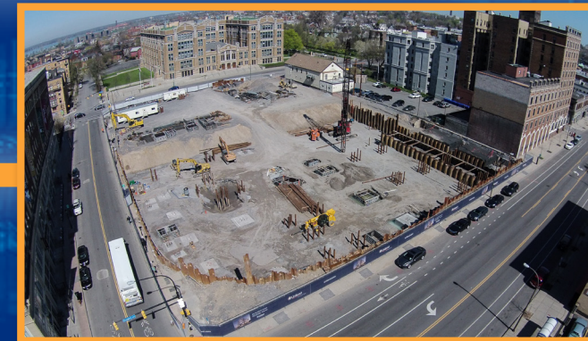
May 11, 2014: Site is cleared and the foundation is installed
