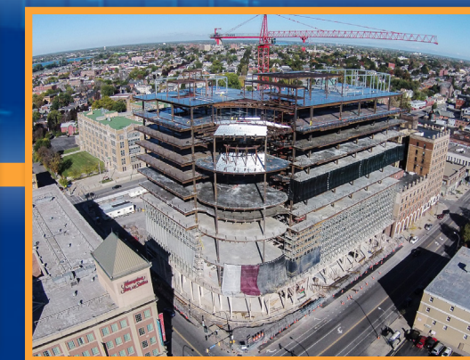
July 18, 2014: Erecting the structural skeleton
