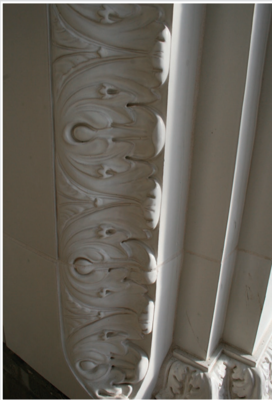
Detail of new terra cotta custom fabricated by Boston Valley Terra Cotta and installed by expert masons
