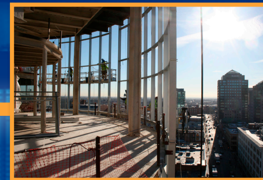
March 19, 2015: Crews prepare for glass installation
