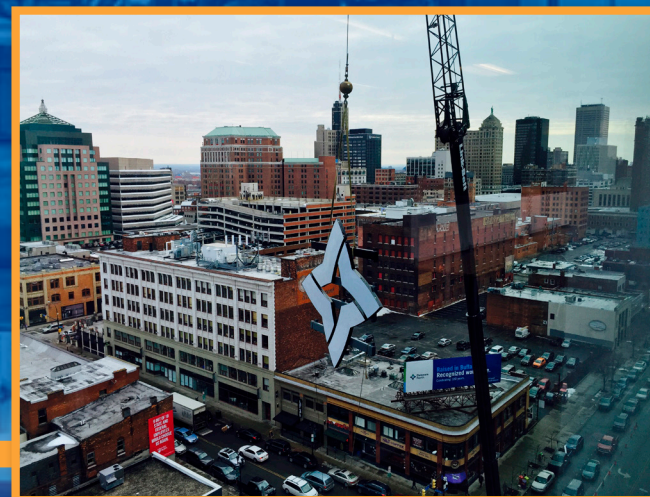
January 28, 2016: Part of Delaware North's sign is raised for installation to the top floor. The sign is white during the day and, at night, the star portion of the sign displays the company's brand colors
