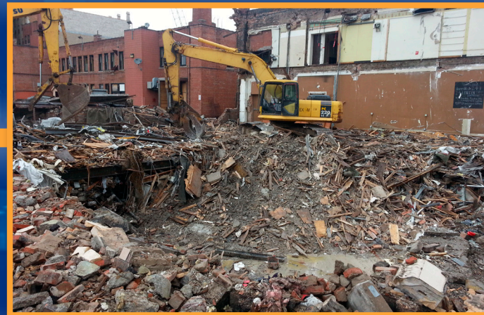
March 19, 2014: Deconstruction of the former Delaware Court
