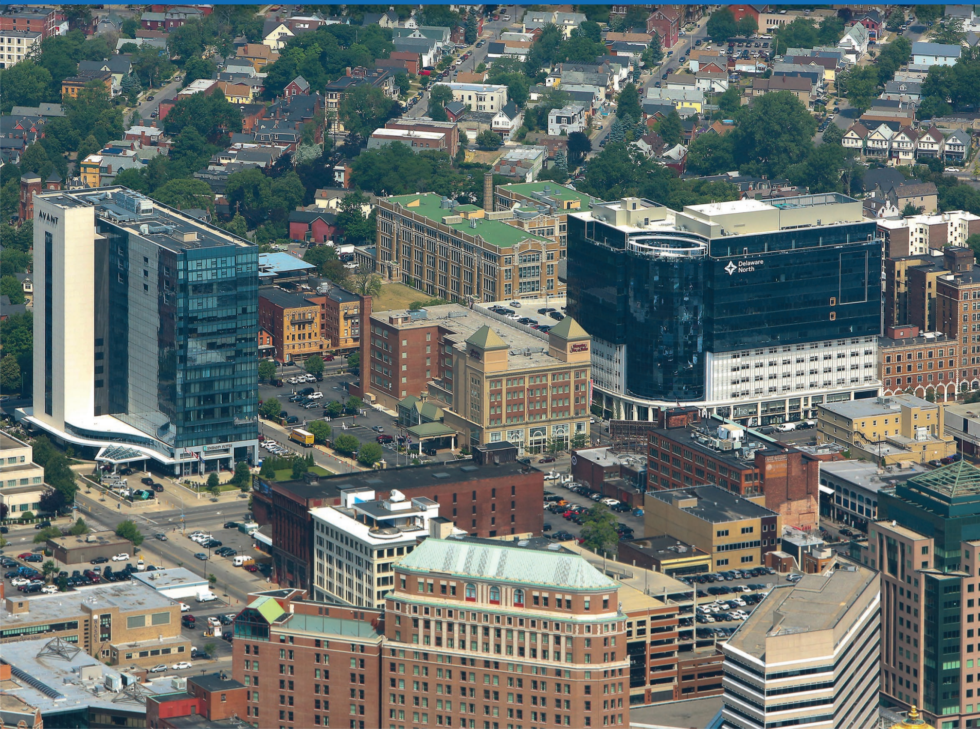
Uniland's latest developments on Delaware Avenue in Buffalo
