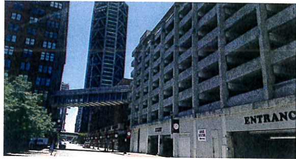
7th Street Parking Garage
