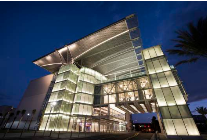
› Exterior View of Dr. Phillips Performing Arts Center
